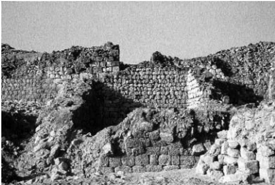
Fig. - 13 Northern side of tower.
