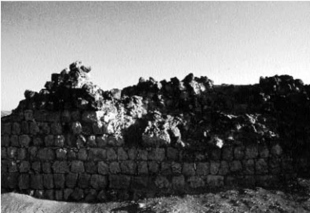
Fig. 12 - City gate. Northern side of the external barrier.
