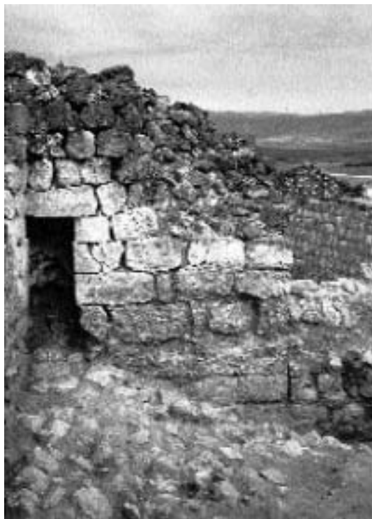
Fig. 10 - View of the area A7, with the postern's exit.
