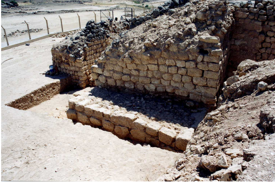
Fig. 5: City Gate. The foundation of the old tower A47 and the western side of later smaller tower (A9-A2). The towers are built with gigantic roughly hewn stone blocks with the body” of small and medium size unworked stones.
