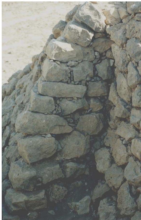
Figura 12: , corner of the city-wall M25 during consolidation
