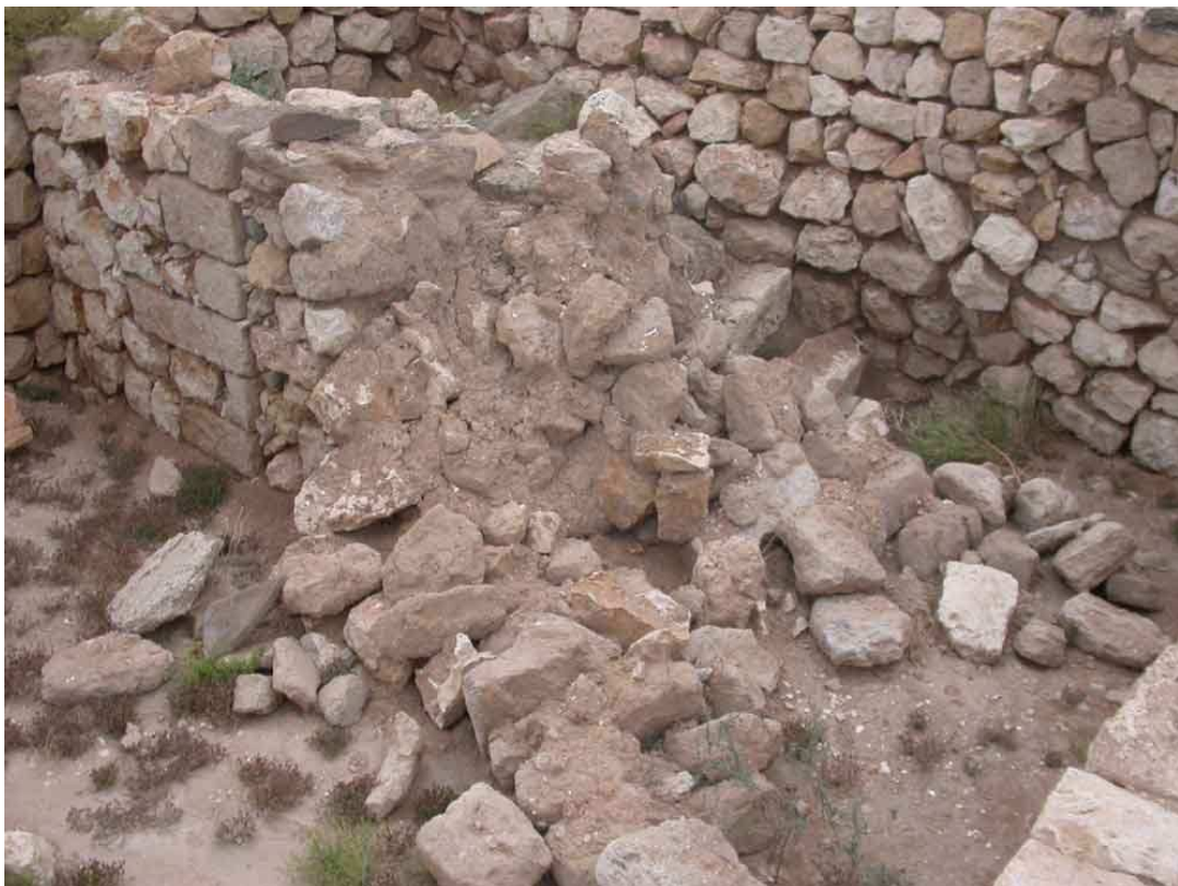
Wall M56 after the rains and before restoration
