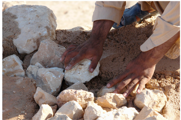
M223 – Top beautification: once the wall is finished, a sloping layer of mortar is bedded with different sized stones on top and filled again with the same type of mortar used for the wall front.
