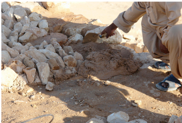
M223 – Top beautification: once the wall is finished, a sloping layer of mortar is bedded with different sized stones on top and filled again with the same type of mortar used for the wall front.
