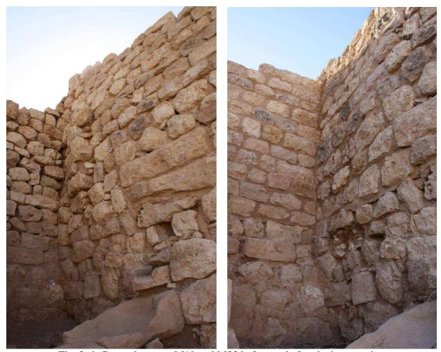
Fig. 2a,b Corner between M19 and M23 before and after the intervention
