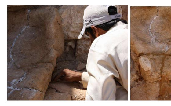
Figs. 8-9 Filling of the cracks and of the basement
