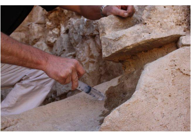
Fig. 5 Injection of Paraloid solution at 3%
