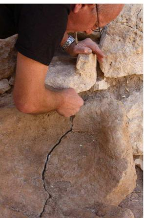
Figs. 6-7 Preparation and placing of the restoration mortar
