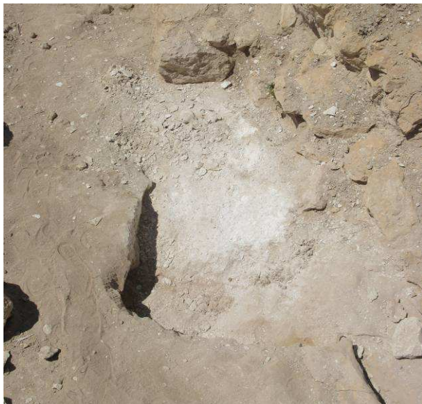
Fig. 2 Chiseling the bedrock for the placement of the foundation blocks.
