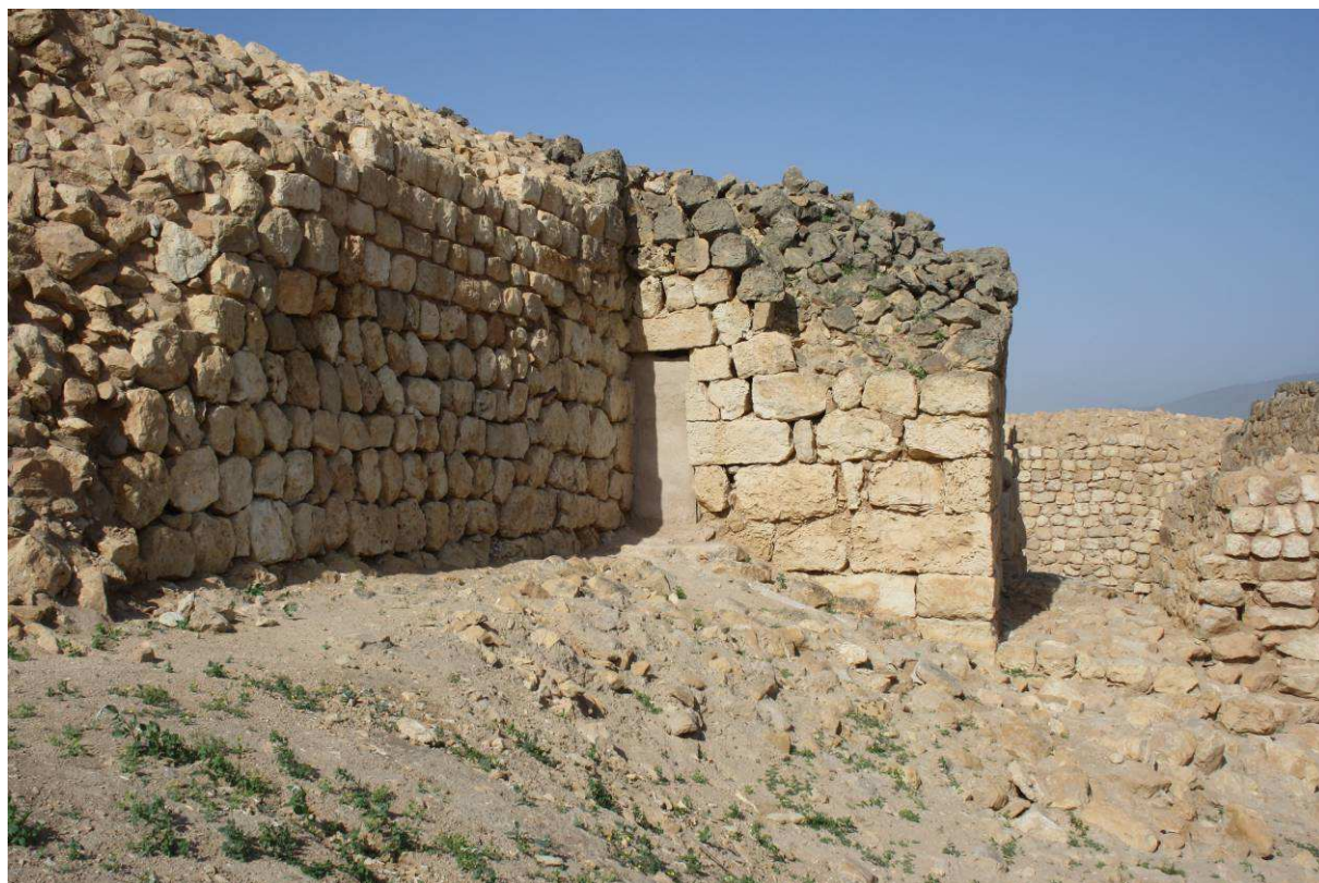
Fig. 3, the postern gate after the placement of the mortar covering
