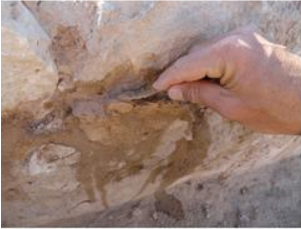
Laying of new plaster
