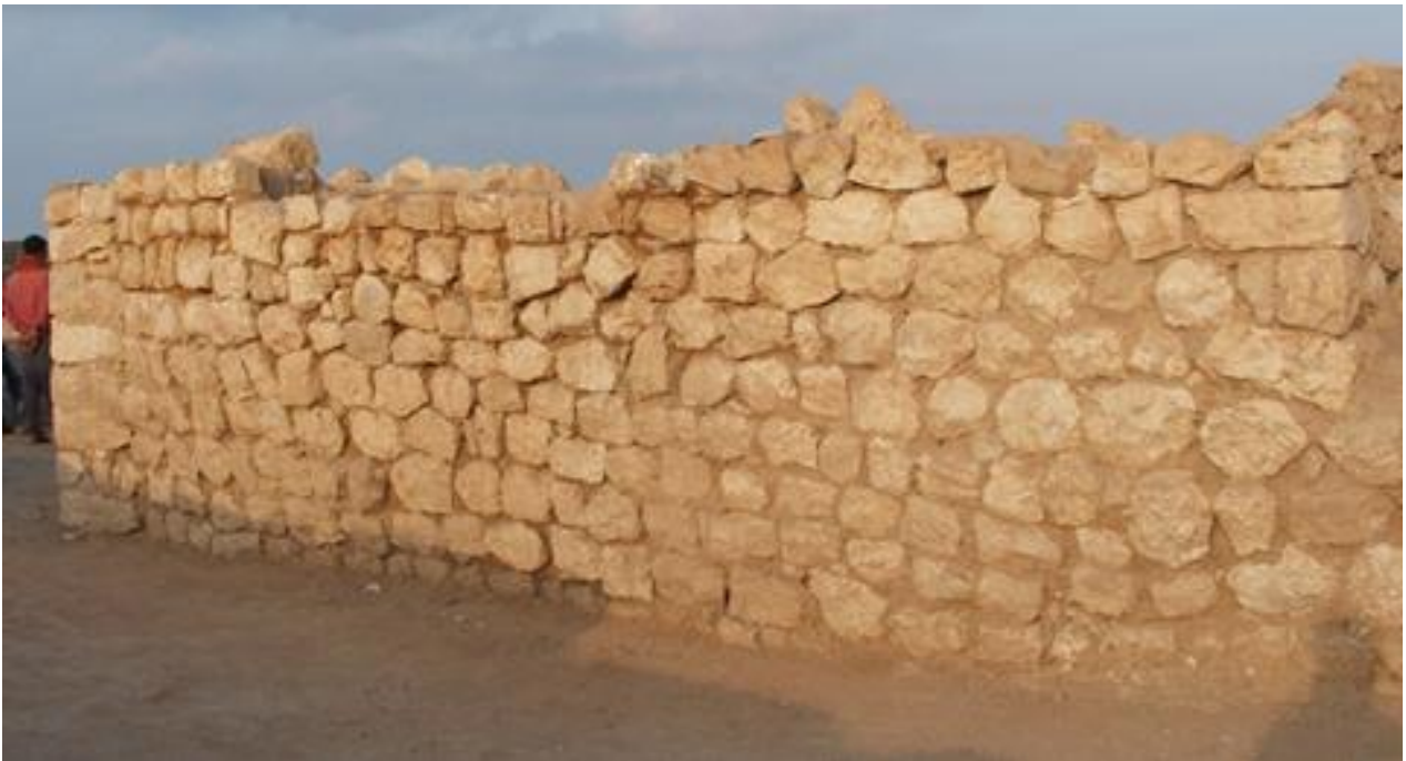
M484, east front wall, after the restoration.
